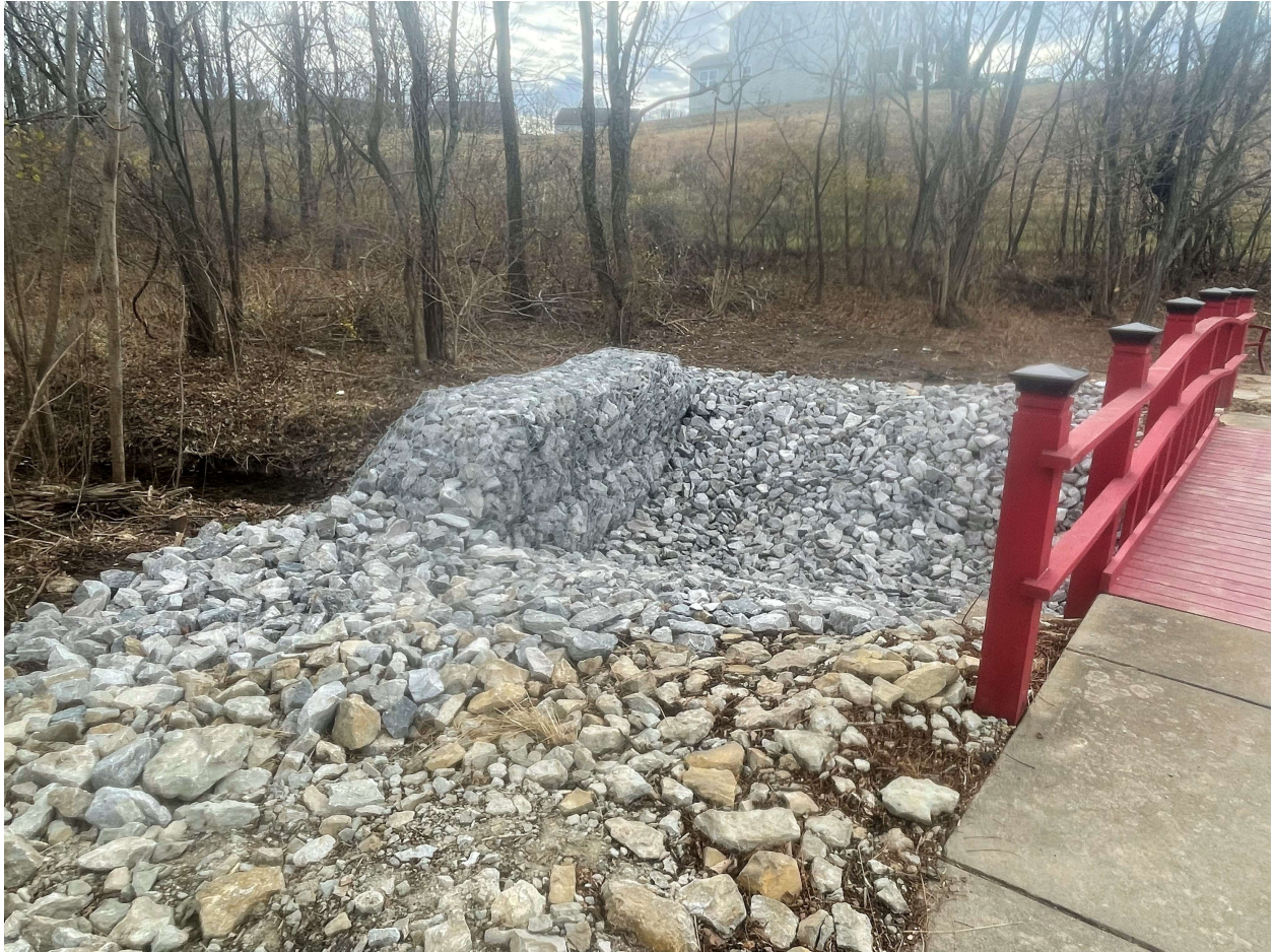
A nearby check dam they did in Union if anyone wanted to check it out. Harmony HOA. Location is below.
